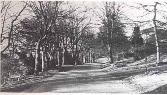
LINCOLN ROAD FROM WOODSIDE
