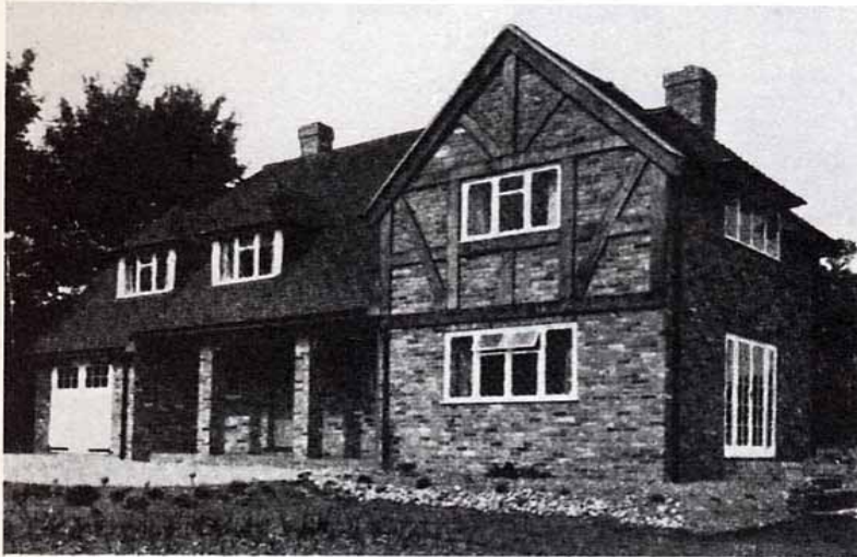
This house in Ellis Avenue, Chalfont St. Peter, faces south-west, and stands on a rectangular plot 65 ft. by 175 ft. Plans are included in an article about the estate beginning on page 177.
